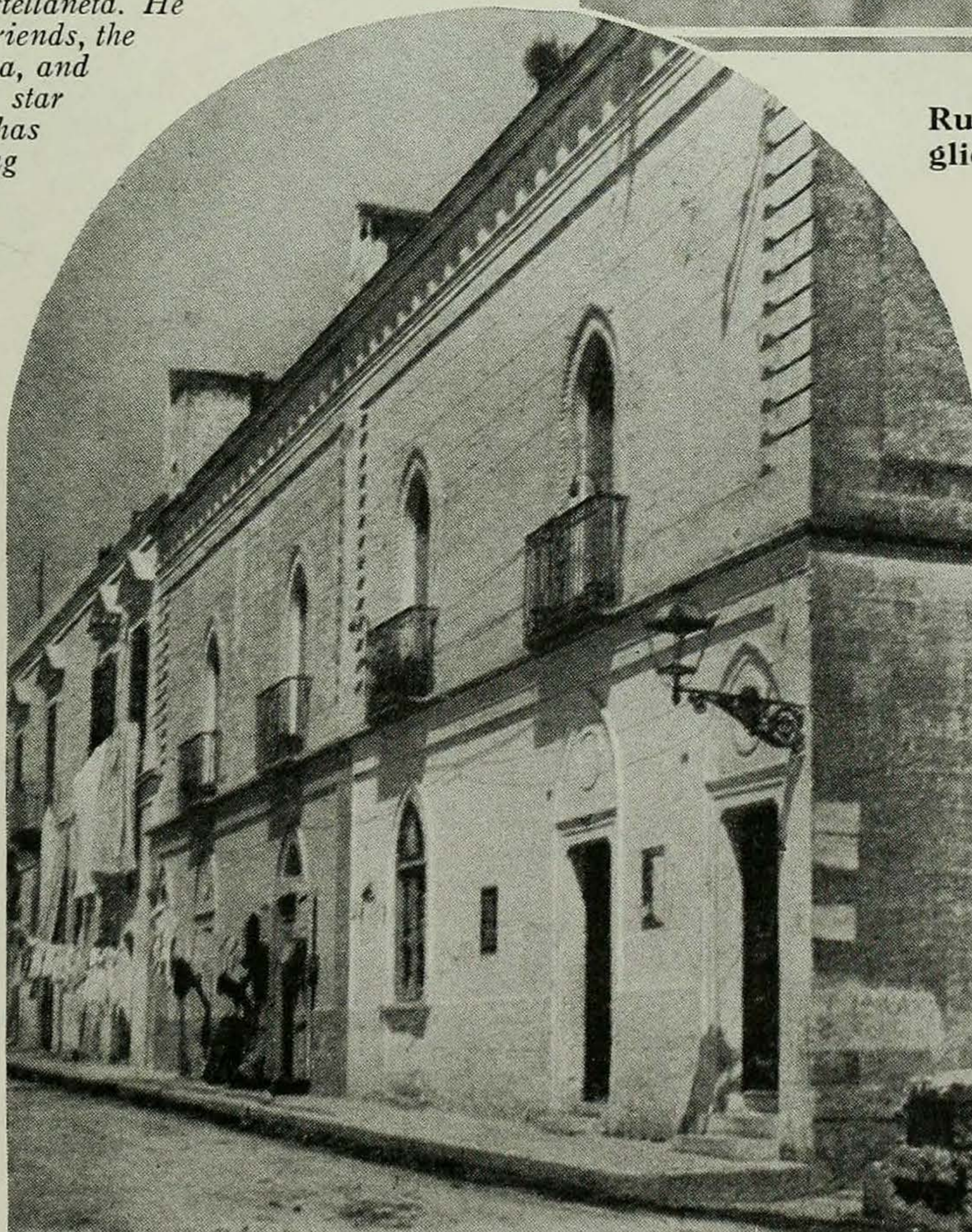
Valentino was born in the small room above the door of this white corner house
